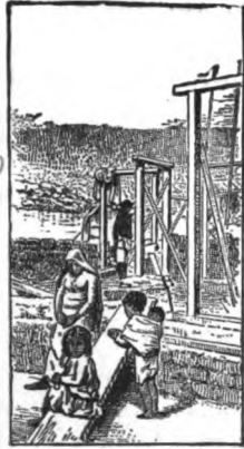
Building the hospital.
