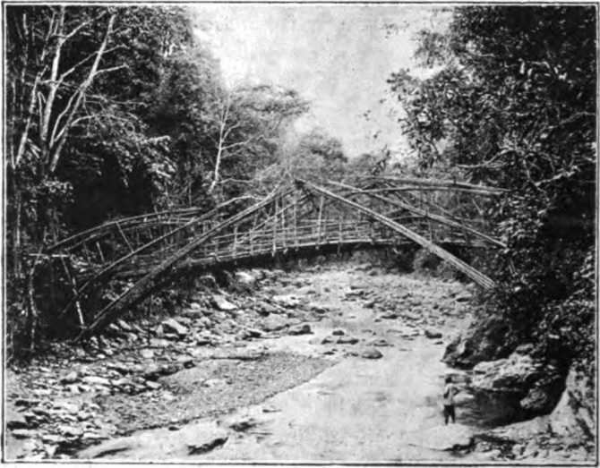
A broken bridge.
